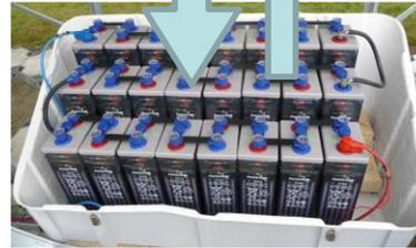
Deep Cycle Batteries provide continuous DC power.
