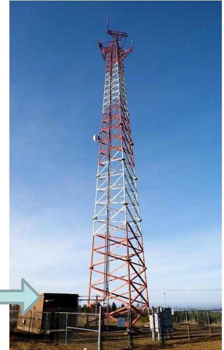
The Tower BTS needs 48V DC at typically 2kW.
