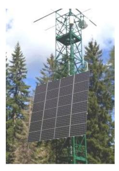
4) This PV Array is hung from the tower by a hinge at the top edge of the array. Then the bottom will be pushed out with struts to the proper tilt angle.
