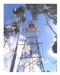
7)This photo taken from below shows the PV Arrays at 3 different levels. The frames extend beyond the sides of the tower.
