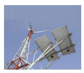
5)A tiny version shows a simple 2 module array off the sides of a tower. This would work at, or near the Equator, but many more PV modules will be required.
