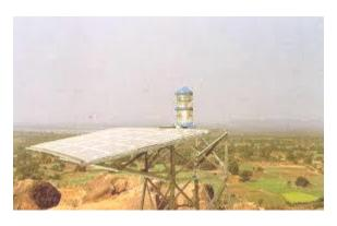
3)This is one form of ultimate solution to avoid shadows near the equator. The PV Array is mounted at the very top of the tower. There are 20 PV modules. The telecom antennas and microwave backhaul dishes are below the PV array.
