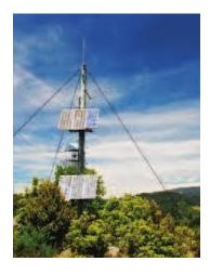
6) This is a guyed pole antenna, and the PV Array is mounted to the pole in 2 tiers with 6 modules per tier. In this case they are above the trees to avoid shade.
