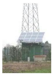
1) This site simply lifts the PV Array as high as possible above the shelter and other equipment inside the fence. This way, the only two things requiring space on the ground inside the fence are the PV array and the tower itself.
