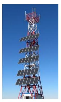
8)This is the ultimate example of mounting PV modules on a tower. There are 5 groups of 6 PV modules mounted at different levels for a total of 30 modules. From the angle of the modules we can guess that the tower is located at above 30 degrees North Latitude, but the principal is the same at any latitude.
