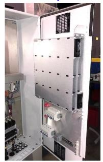
The Rectifier Shelf is mounted on the door. The compact system supports up to 7 of our 3kW SMPS modules plus the Controller. Easy access is provided to the Circuit Breakers and ATS mounted below the Rectifier on the door
