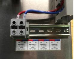
The PV inputs have screw type connectors which will accept up to AWG 2 wires from the Combiner Boxes. <u>Torque the screws to</u> <u>4.6 N-m (40 in-lbs).</u>
