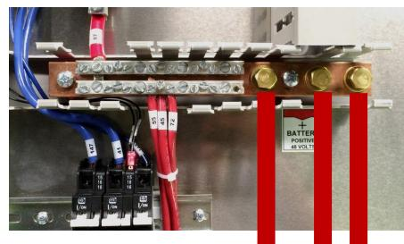
The POSITIVE battery cables are to the POSITIVE BUS BAR.
