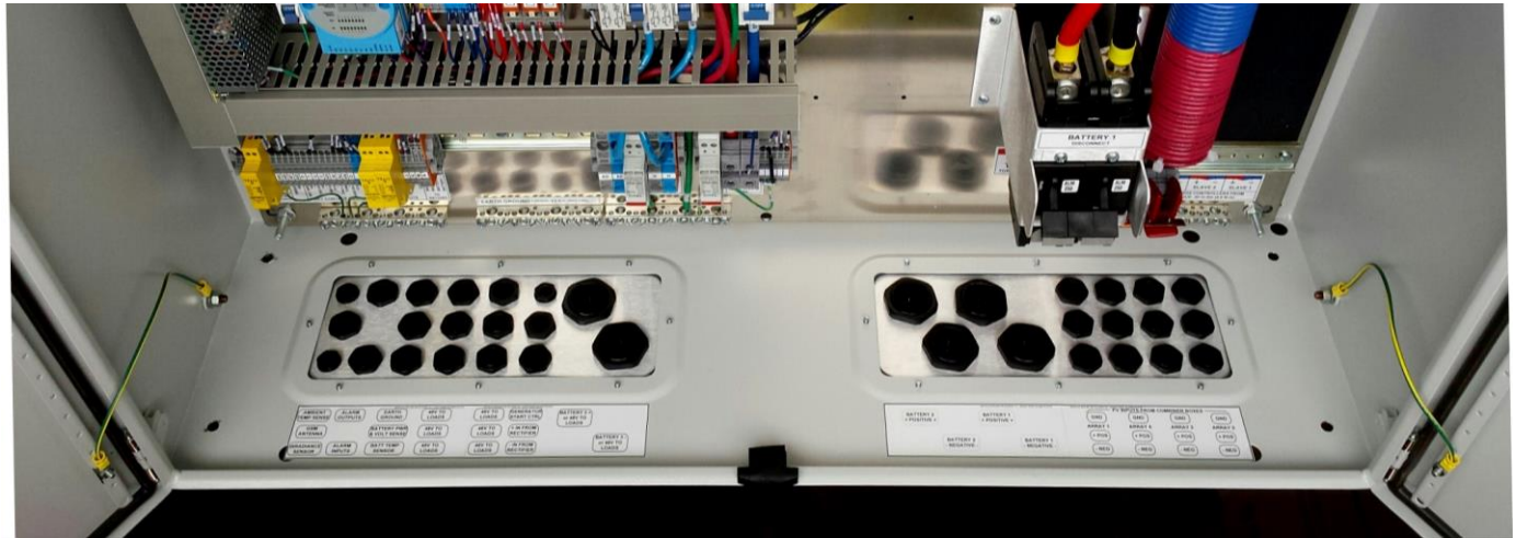
Left and Right side Gland Plates with labels at bottom of Cabinet
